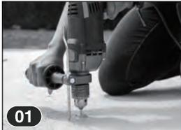
**01** Drill 4 holes in on the surface according to the size as base dimension shows.
